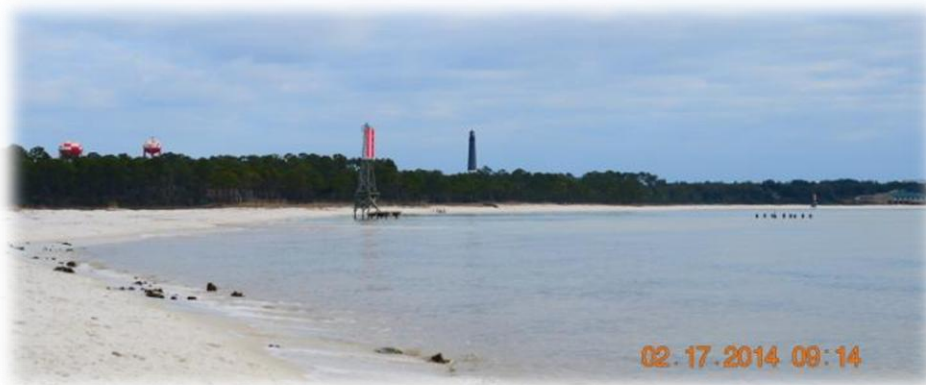
Conditions at NAS Pensacola
